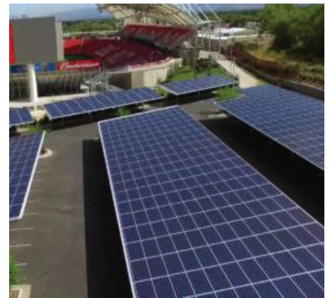
Parking Lot with (Solar Panel) Covered Parking
