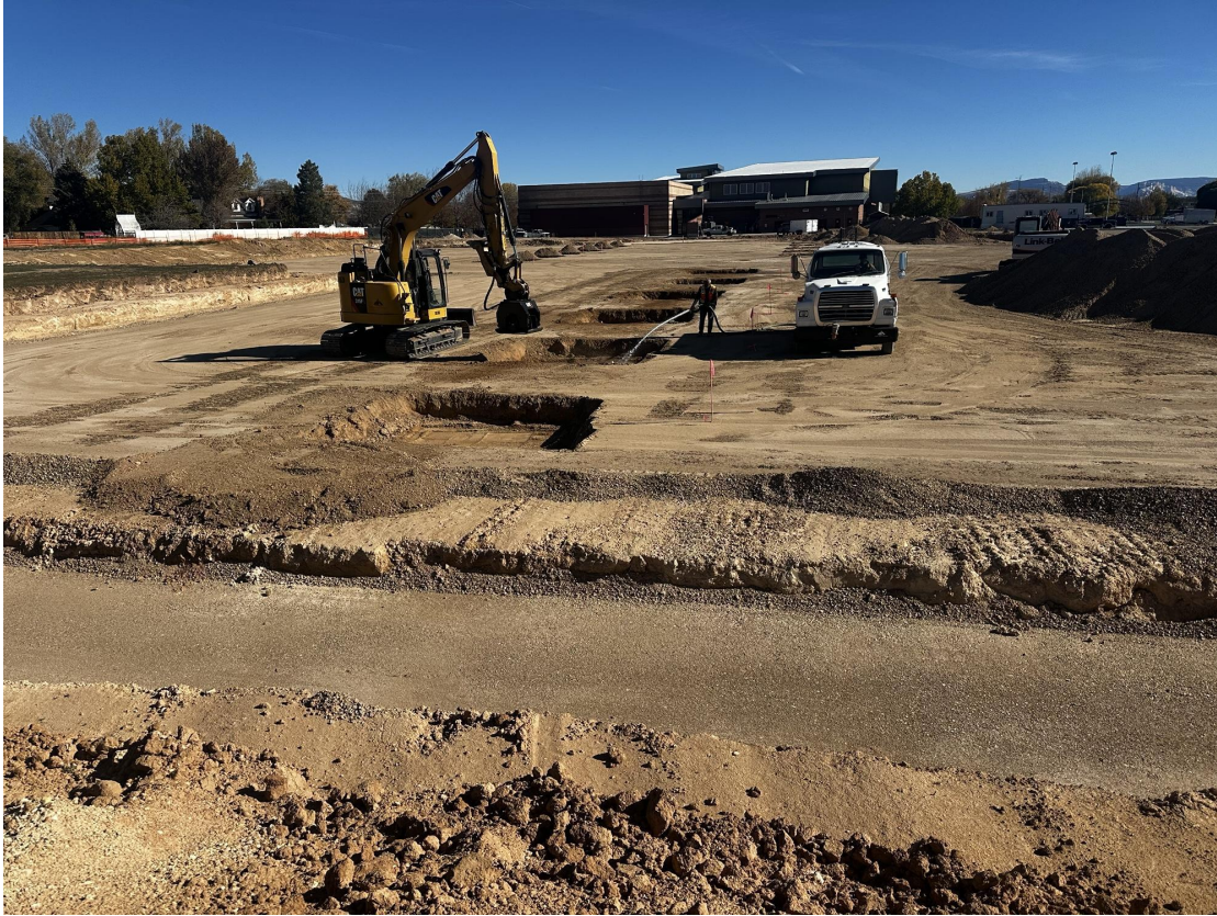
Footing and Pad Prep
